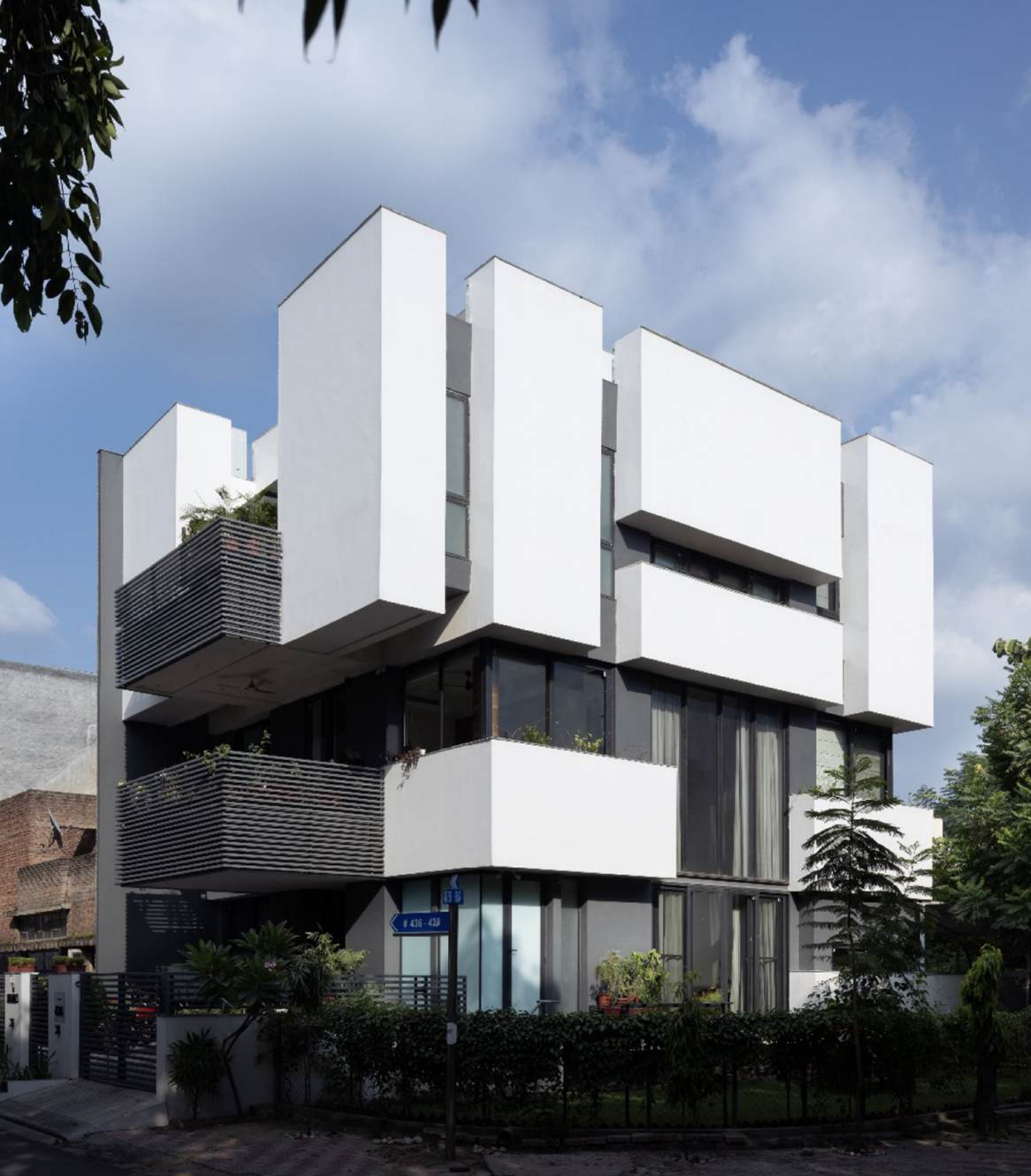
From a 45-degree view, Lacuna House reveals its thoughtful geometry and restraint. Positioned on a corner plot, the house takes full advantage of light and ventilation from both sides.
